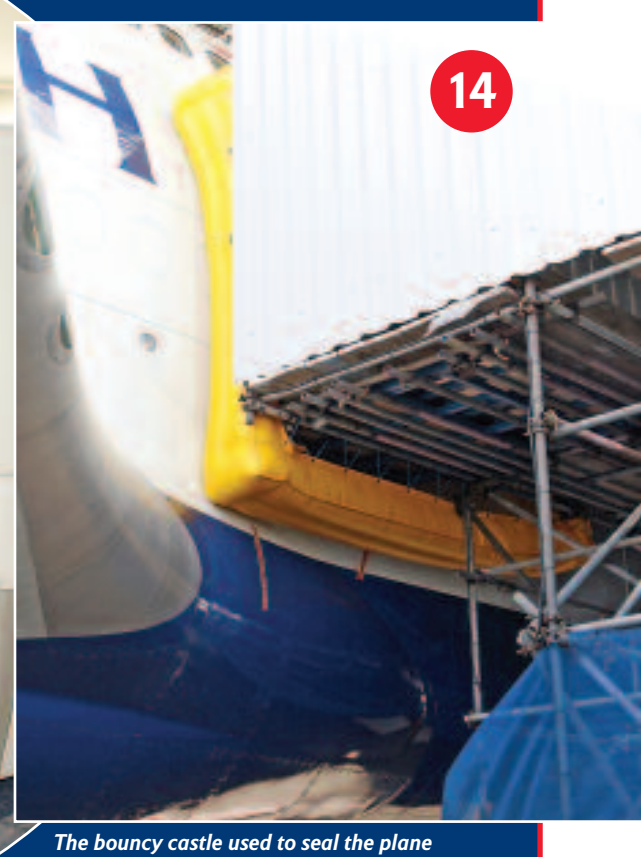
The bouncy castle used to seal the plane during fitting
