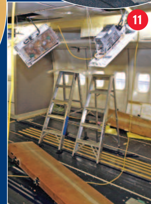
Cabin with old seats stripped out ready for fitting new ones
